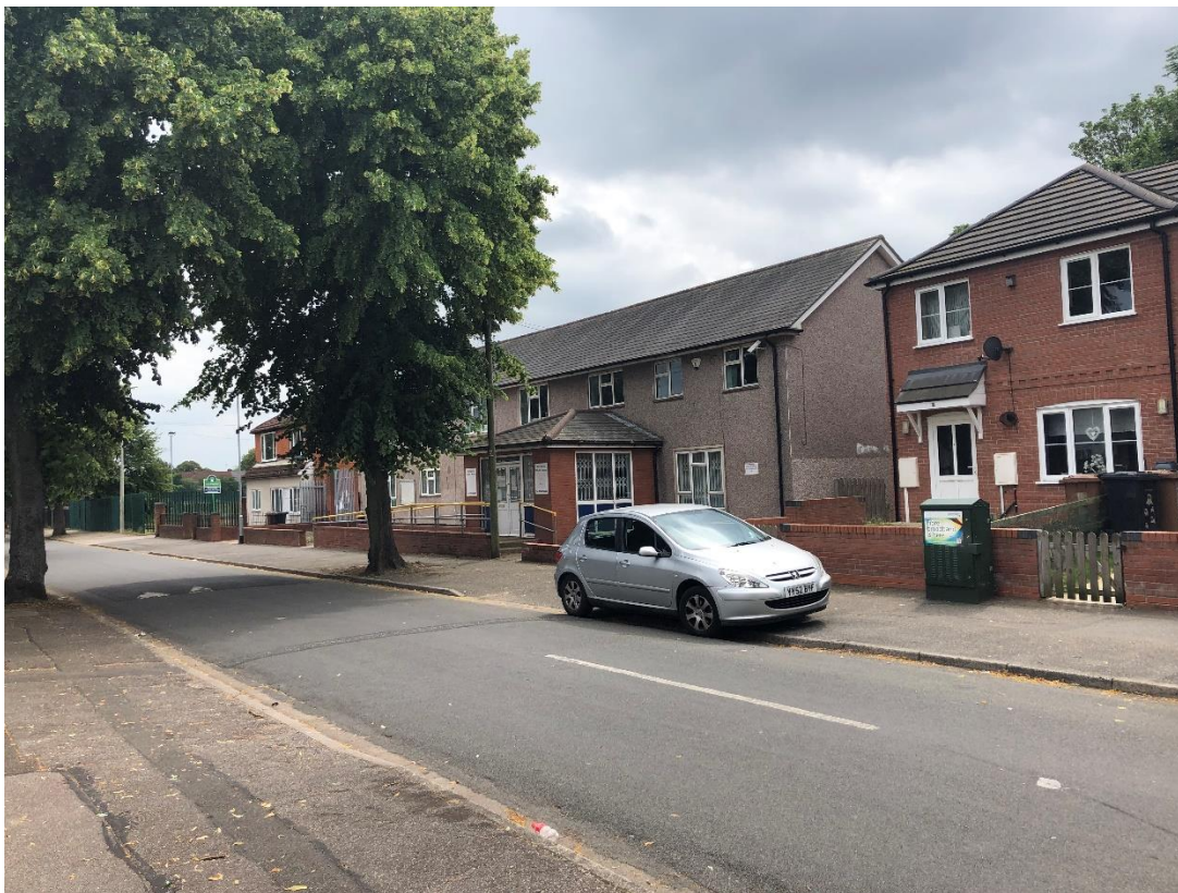
77 Swift Gardens to the right of Markham House with highway tree to front
